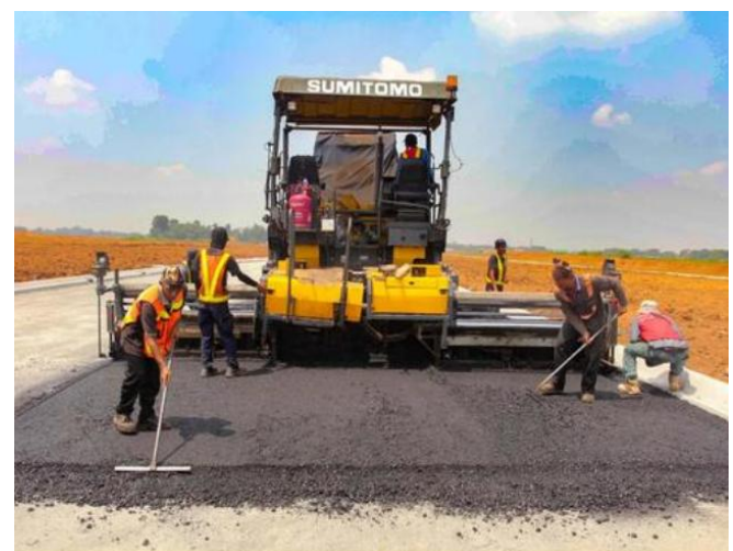
Figure 5. Construction of Plastic/Rubber Modified Road
